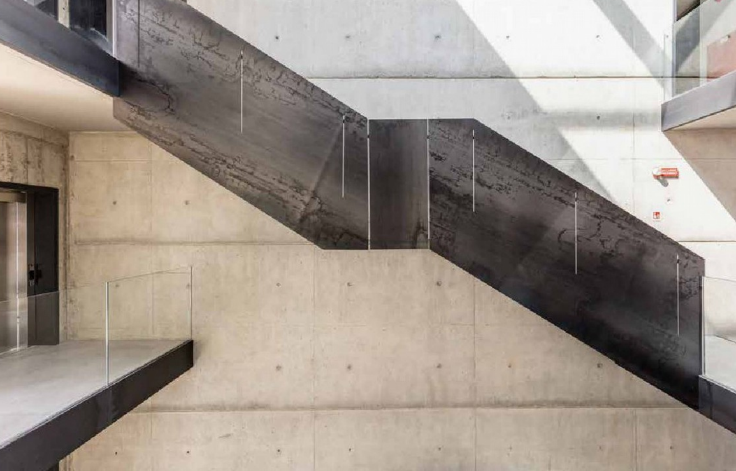
Paint application carried out on site in black iron effect.
